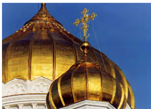
Fig. 6.8 Cathedral of Christ the Savior (Moscow), stainless steel with decorative and protective titanium nitride (TiN) coating. (For a full color version of this figure, see the Color Section)
