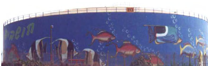
Fig. 6.15 Anti-corrosion protection as well as decoration of a storage tank (Israel).
