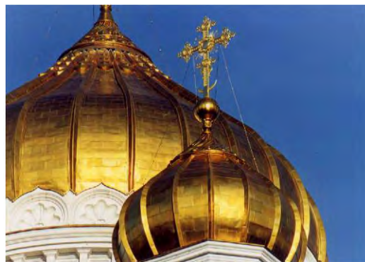
Fig. 6.8 Cathedral of Christ the Savior (Moscow), stainless steel with decorative and protective titanium nitride (TiN) coating.
